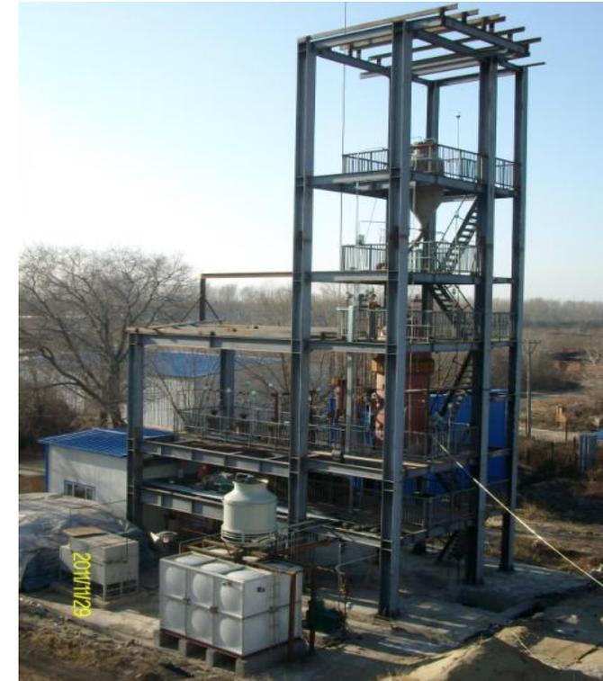
1.2t/d Pure Oxygen Compression Coal Dust Gasification System
